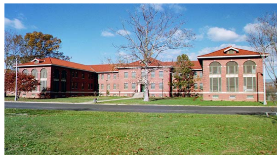
Building CT8 - Treatment Mall Photo by Jogues Prandoni
